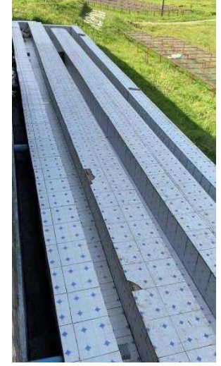
Narrowed Grading canal
