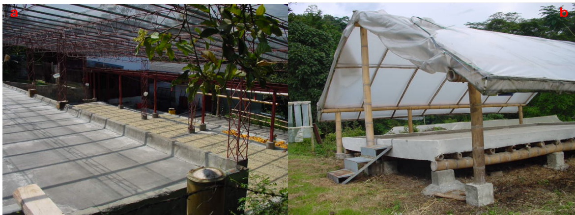
Fig. 3: a. The marquesina is typically constructed in steel and glass so is expensive; b. The parabolicos was designed to be built with local materials such as bamboo, and is aimed at smallholder farmers.
